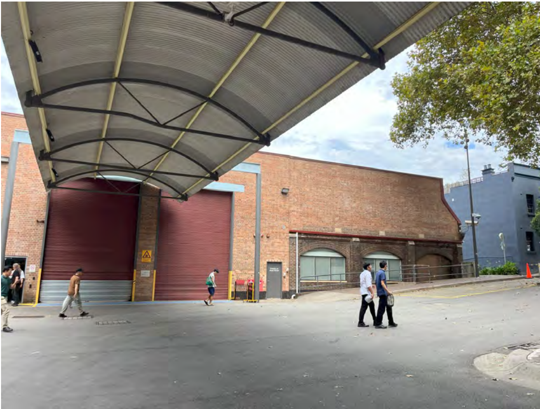
Figure 26 North elevation of the Harwood Building
