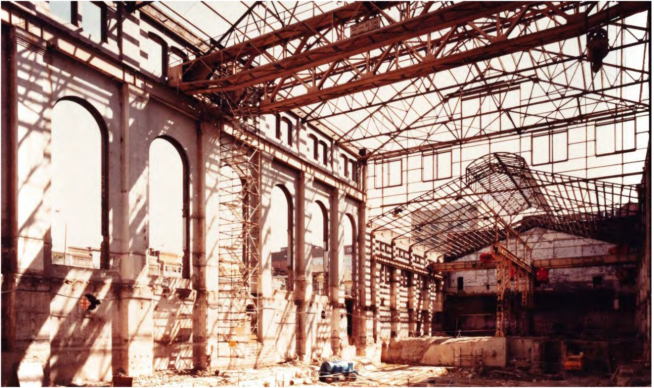
Figure 13 View looking north from the Turbine Hall, during adaptive works (1980s) Source: Powerhouse Museum
