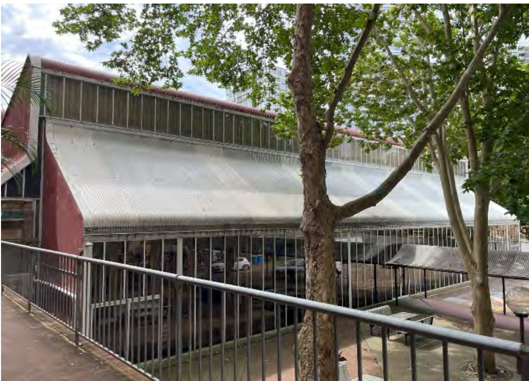
Figure 25 The south elevation as seen from Omnibus Lane
