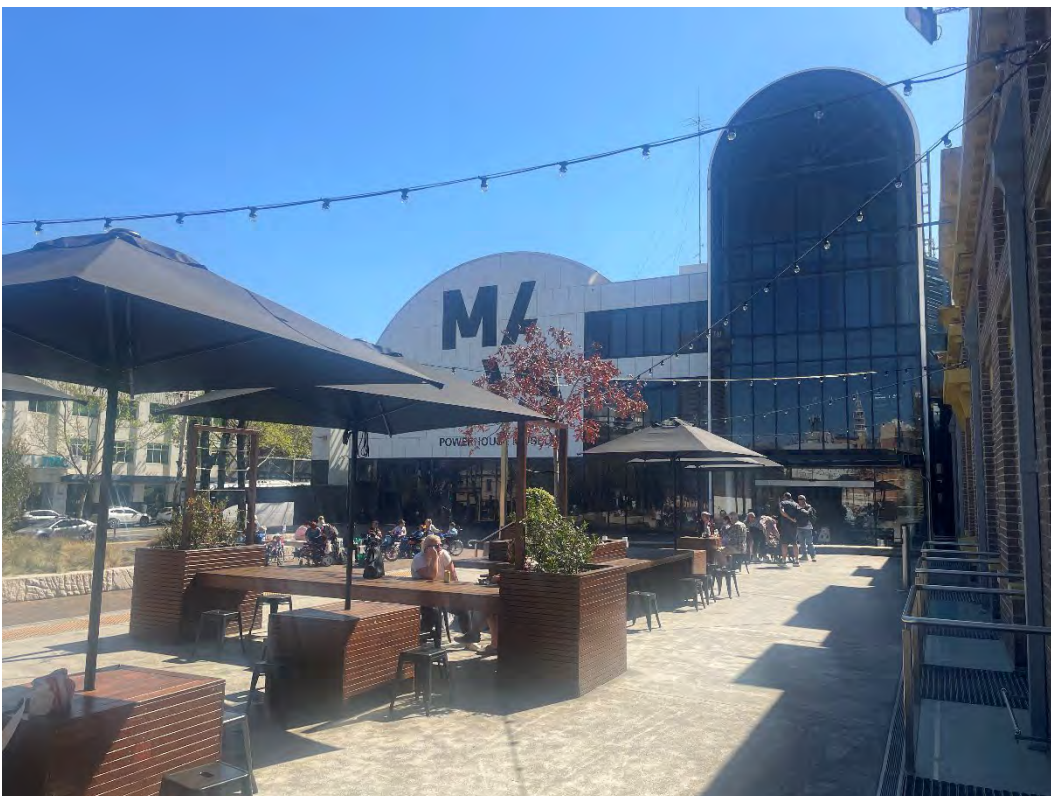
Figure 41 View looking towards the Wran Building from the platform outside the Switch House (September 2023)
