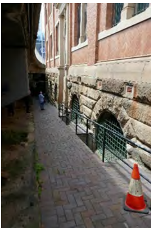
Figure 8 Paved laneway to the north
