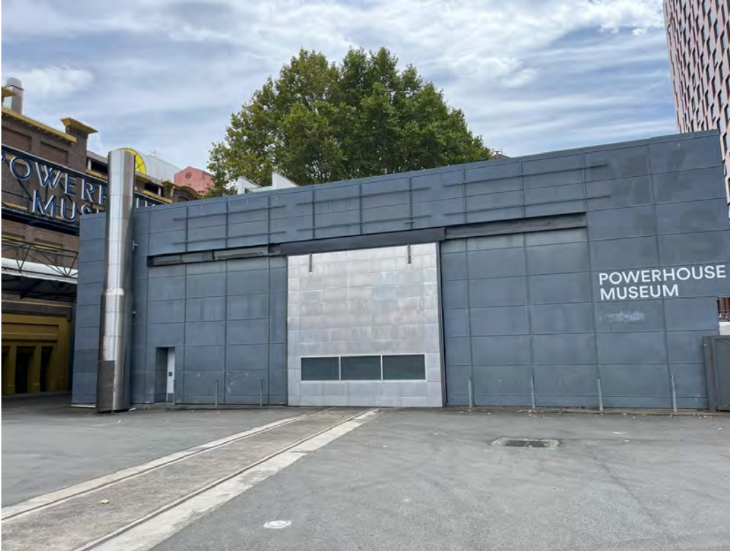
Figure 45 South elevation of the café
