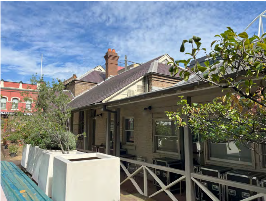
Figure 16 Rear (south) elevation of the 1980s addition (right) and the 1900-01 buildings (left)
