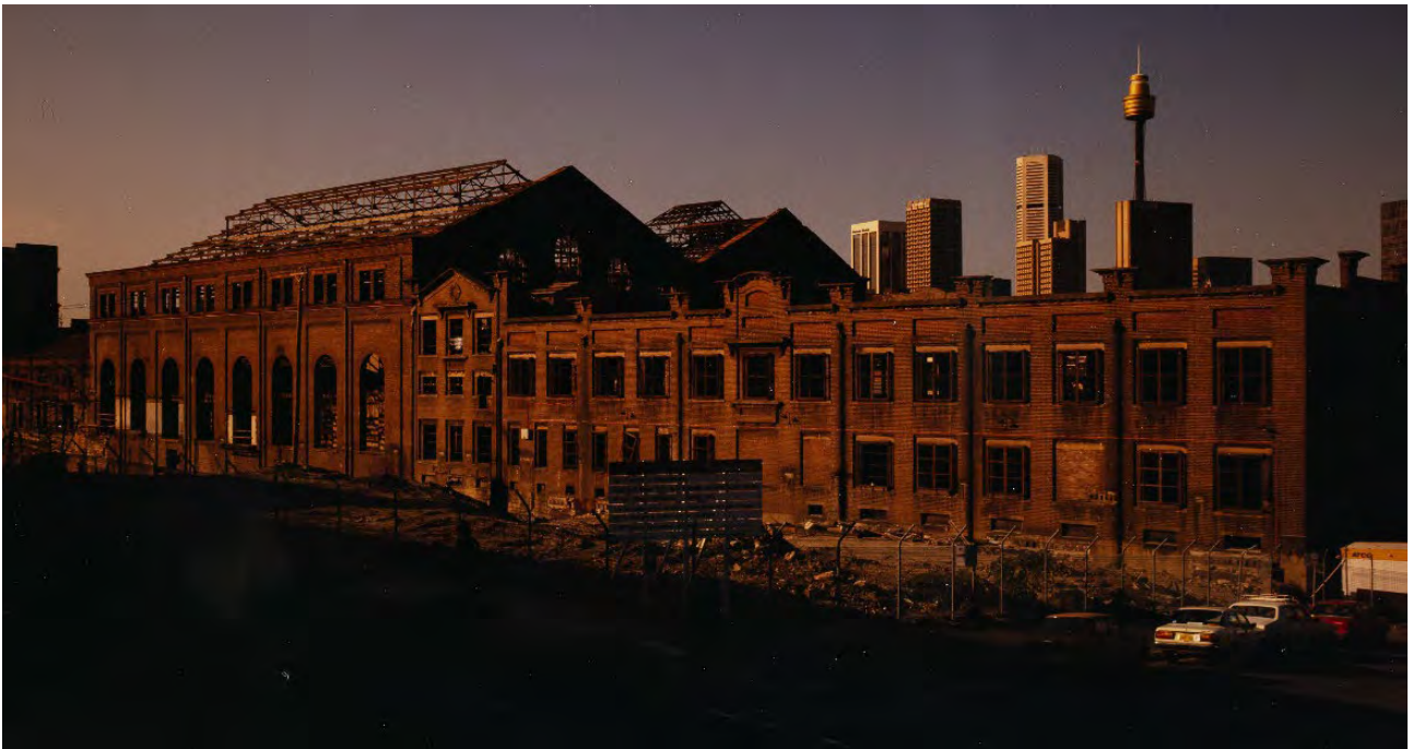
Figure 14 View of the Power House looking northeast (1980s) Source: Powerhouse Museum
